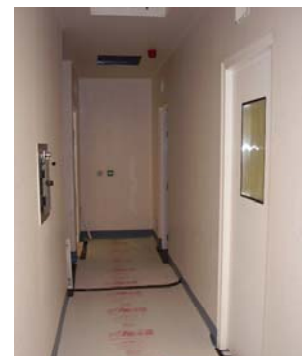
2. Progress on 16 Oct 06
